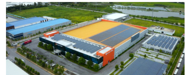
Solar panels at the Vietnamese subsidiary
